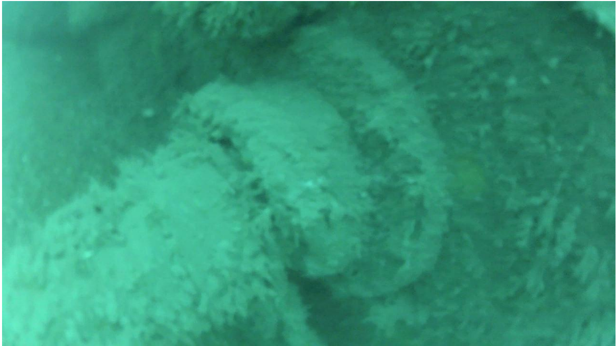
Photo 24, Close up of bearing seen in Photo 22.
